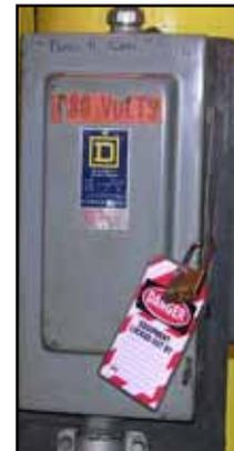
4. Attach a lock and tag that meets OSHA requirements for lockout/tagout to the electrical service entry panel.
